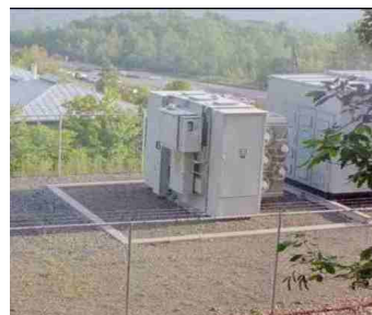
Transformer with Automatic Load Tap Changer
